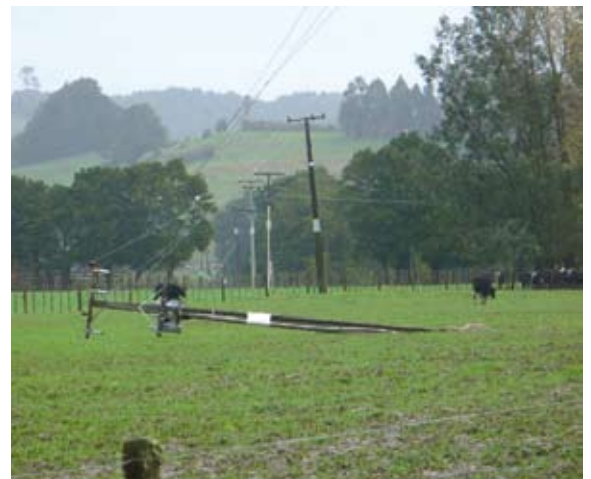
The storm caused more destruction than Cyclone Bola
