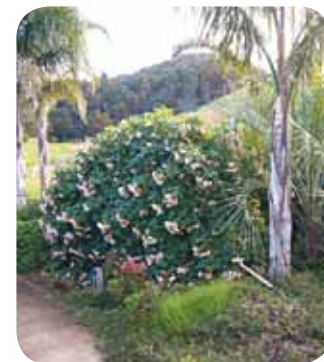
Can you find the transformer box?
